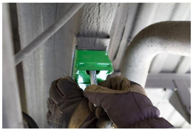
22) Since there is groove where the mounting holes land, a step drill will need to be used for drilling. Center punch the hole locations and drill with a step drill bit to a diameter of ¼" (7mm).
