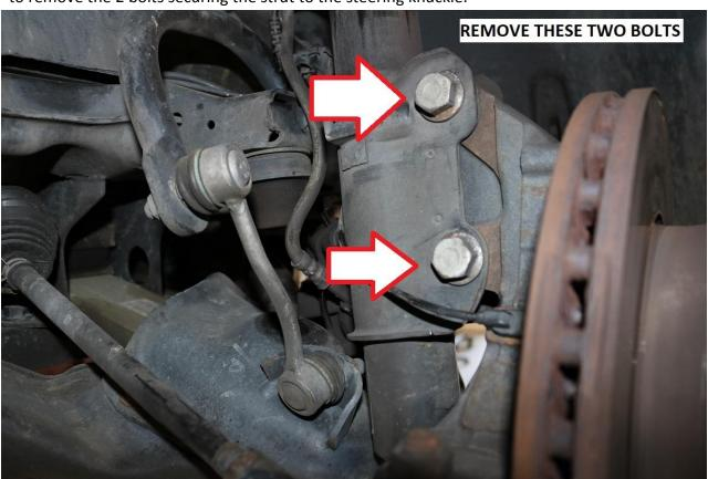
22) With the strut disconnected from the steering knuckle, allow the lower control arm to hang free again. Be careful to slowly lower the knuckle out of the strut. Be sure the wheel speed sensor wire is not strained.
