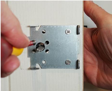
3. Remove the two screws that holds the keyed cylinder in place. Leave the back plate in place. Keep the screws .
