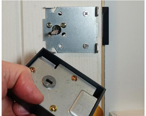
2. On the inside of the door, remove the nightlatch. It is usually secured by two screws.
