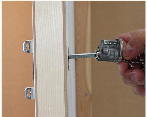
4. Remove the keyed cylinder from the door. Keep hold of the ring.
