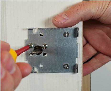
9. Fix the cylinder in place with the 2 existing screws and tighten.
