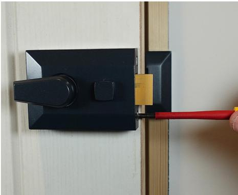
11. Secure the latch using the 2 screws.
