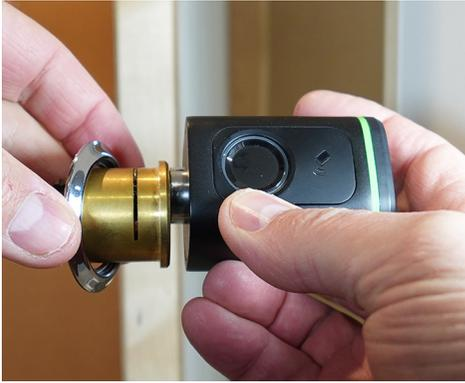
7. Install the existing ring over the brass cylinder.
