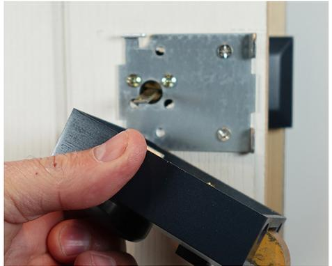
10. Refit the latch on to the backplate.
