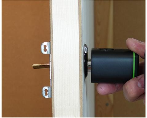
8. Push the lock handle through the door. TIP: Hold in place with masking tape.
