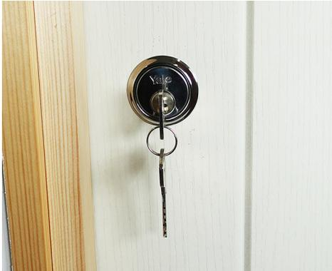
1. This shows the existing nightlatch keyed cylinder. This is the part that will be replaced.
