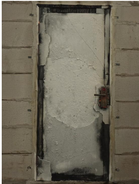
Fig. 6 Exposed Side after 60 Minutes
