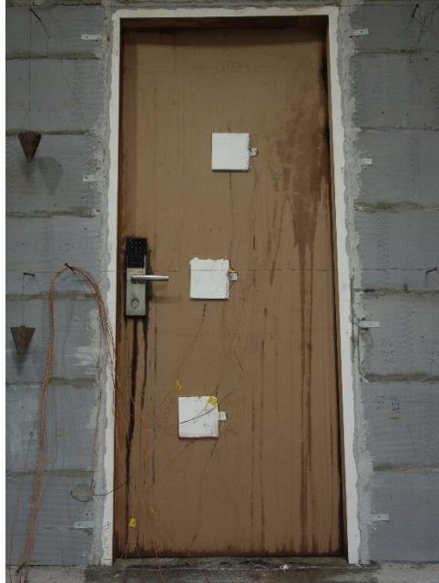
Fig. 9 Unexposed Side after Hose Stream Test
