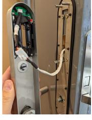
STEP 15 Offer up the internal handle and connect the cable to the battery pack via the white plug.
