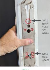
Apply masking tape to both sides of the door. Insert the spindle back through the latch. Draw a line at the spindle centre and extend horizontally and vertically both sides of the door. Remove the backplate from the inside lock body and align on the door like this. Mark the
