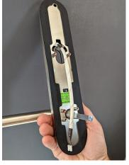
STEP 10 Fit the rubber gasket to the rear of the front lock body.
