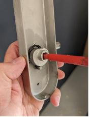
STEP 8 Check that the handles are facing the correct direction. If not insert a Phillips screwdriver, loosen the screw fully, turn the handle 180 degrees and then tighten the screw. IMPORTANT: Even if the handles do not need reversed, insert a screwdriver and fully tighten the screws.
