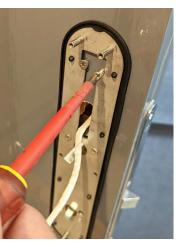
STEP 14 OPTIONAL: We recommend fitting two additional screws to hold the backplate flat to the door like this.
