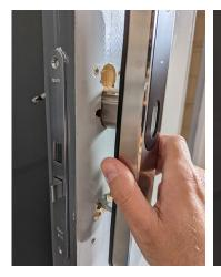
STEP 11 Offer up the external lock body, aligning the spindle through the mortice.
