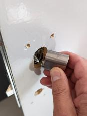
STEP 2 Remove the existing keyed cylinder and keep for later.
