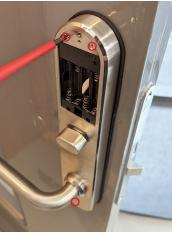
STEP 17 Using the 3 short screws, secure the lock body to the backplate. Make sure that the body fits within the rubber gasket.
