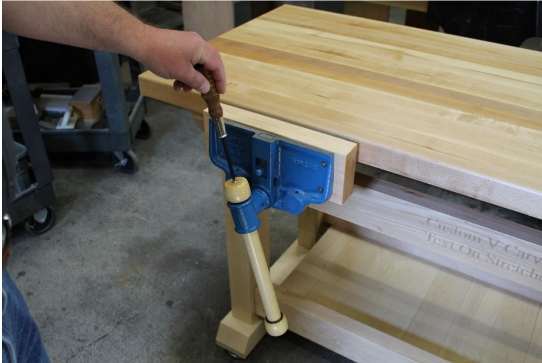
Step 16: Insert and secure the vise handle into place with provided end caps and screws.
