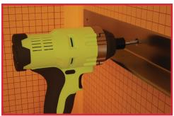
2. Firmly place the bracket against the wall at your desired height and drill through one of the three mounting holes into the kerdi board panel as well as any blocking or studs on the other side.
