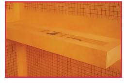
7. Wrap the shelf with the Schluter water-proofing wrap & mud the Kerdi-board.
