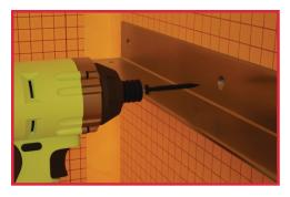
**3.** Switch to the phillips bit and fasten one of the provided screws into your pre drilled pilot hole.
