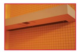
**5**. Fit the notch on your kerdi board to match the width and depth of the bracket.
