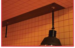
6. Fasten the remaining provided screws to the under mount mounting holes of the bracket.
