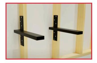
1. Install both brackets at the desired height using the provided hardware. Ensure they are level and securely attached.
