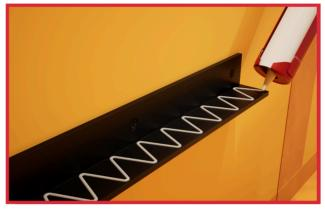
**3.** Apply Kerdi Fix to the brackets and set the first board onto the brackets.
