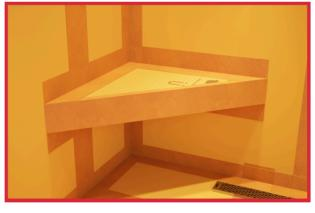
**6.** Apply a layer of thin-set then wrap the exposed sides in the provided Kerdi Band.
