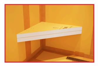
**5.** Place the second board on top of the first board with the Kerdi Fix in between both boards.
