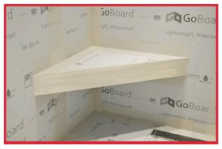
**6.** Apply a layer of thin-set then wrap the exposed sides in the provided tape.
