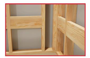
1. Install blocking at desired height between pre-existing wall studs.
