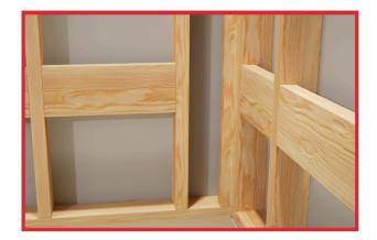
1. Install blocking at desired height between pre-existing wall studs. Apply wall board according to manufacturer specifications.
