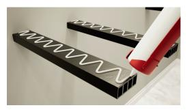
3 Apply adhesive to the brackets, and then set the board.
