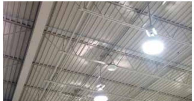
*The corrugated metal roof inside a “Big Box” store. This corrugation allows for the very large roof to have the structure to hold up under conditions like wind, rain, and heavy snowfall.*
