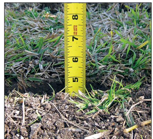
Ensure that dripline depth is consistent throughout the installation
