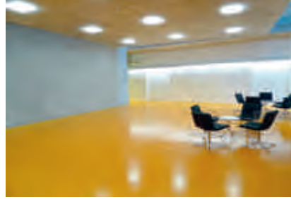
[Fig. 6] Institutes of Pathology and Forensic Medicine, County Hospital, St. Gallen. A PU floor was chosen because it allowed an easy and quick refurbishment, reducing disturbance and increasing acceptance. Silvia Gmür Reto Gmür Architects (I 1) Bild: © cctp.
