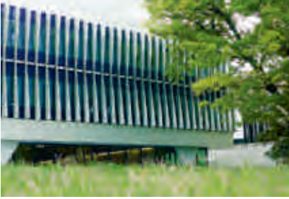
[Fig. 5] Institutes for Pathology and Forensic medicine, county hospital, St. Gallen. Fixed louvers were calculated and designed to reduce mechanism complexity This solution reduces maintenance and disturbance. Silvia Gmür Reto Gmür Architects (I 1) Bild: © cctp.
