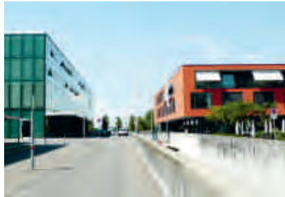
[Fig. 8] Cantonal Hospital Zug and Care Centre. By constructing the facilities next to each other, high synergies are achieved through sharing services, staff, and underground mechanical engineering. Burckhardt+Partner Architects (I 3) Bild: © cctp.
