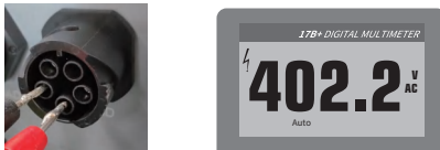
Detecting the voltage between three phases
