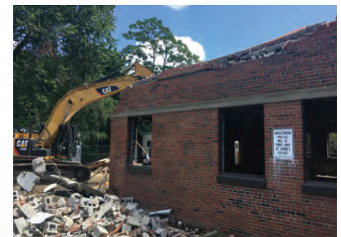
Demolition under way, July 2018
