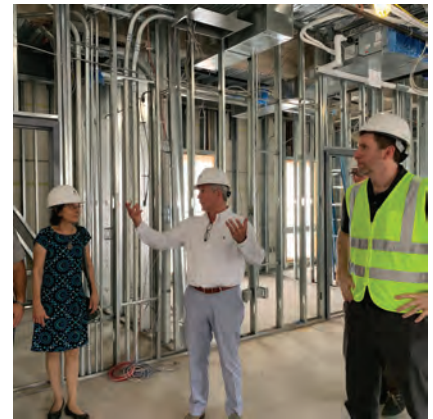
NAASR's new headquarters under construction, August 2, 2019.
