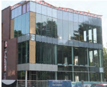
NAASR's new headquarters under construction, August 2, 2019.
