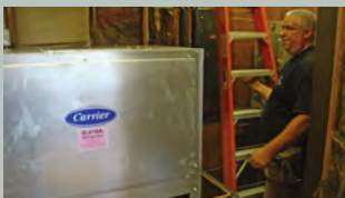
Installation of NAASR's new air conditioning system
