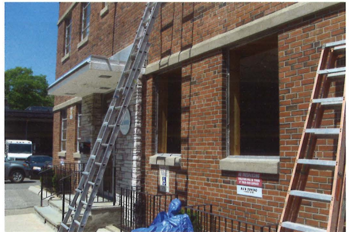
NAASR's new windows being installed in May 2009.
