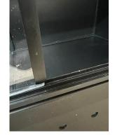
Please note: they are cut to allow for the doors to still be removed while decorating or cleaning so be sure that they are positioned just above the bottom tracks as shown. This should leave you with a  $\frac{3}{4}$  " gap at the top and a  $\frac{1}{4}$ " gap at the bottom when set in place.
