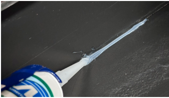
Lay down a bead of silicone along the joints
