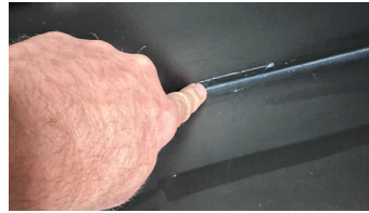
Use a wetted finger to smooth the bead into the seam
