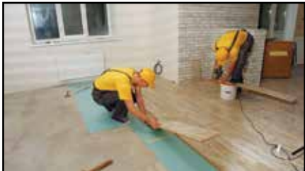
Workers laying down a floor
