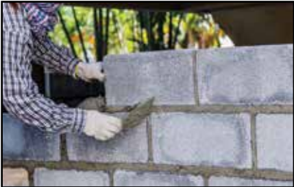
A mason working with concrete blocks for the foundation* of a house
