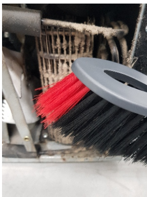
Figure 9: Clean with soft brush or small paintbrush.
