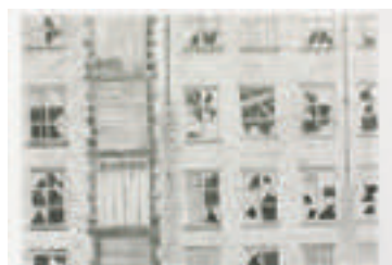
Lot No. 254, Jim Sunderland, Derelict Mill West Yorkshire
