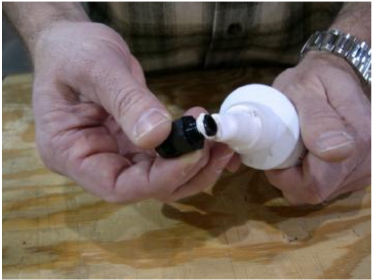
Photo 8. Teflon pipe dope on pipe threads.
