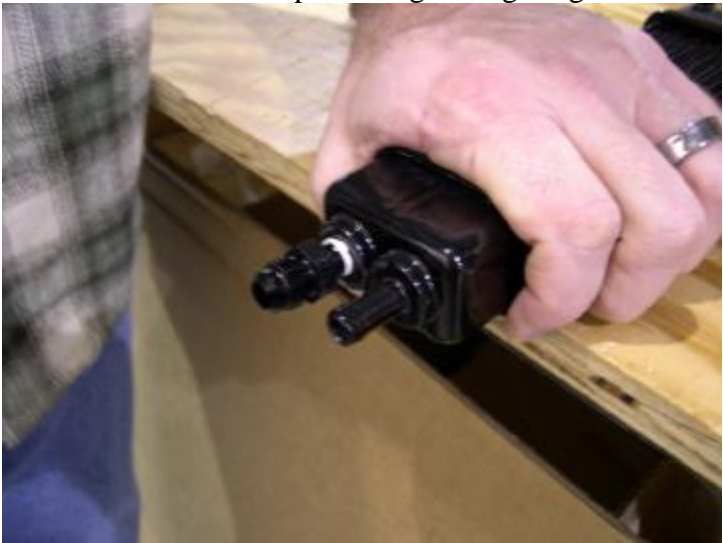
Photo 11. Install 2.5 to 3 times finger tight.
