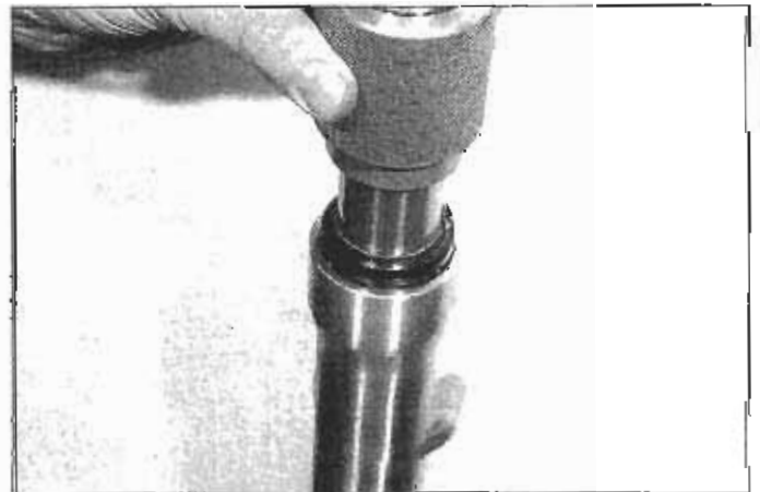
5.27 Use any of the tools previously shown to drive the dust seal into place
