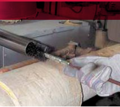
Cleaning boiler pipes with a flue brush.
