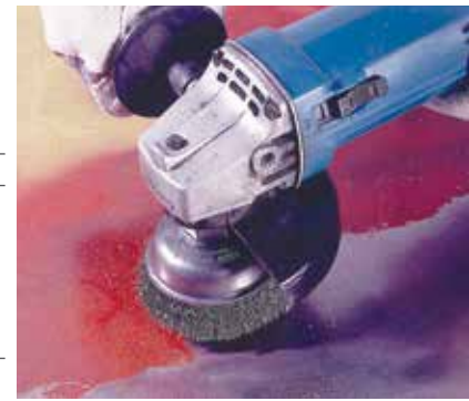
Removing paint from a steel surface with a crimped wire cup brush.
