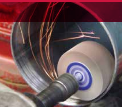
Removing burrs from the inside diameter of a cut tube.
