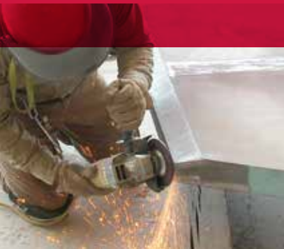
Grinding on a platform for weld preparation.
