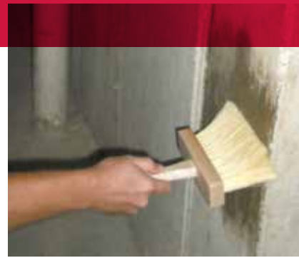
Applying waterproofing material with a masonry brush.
