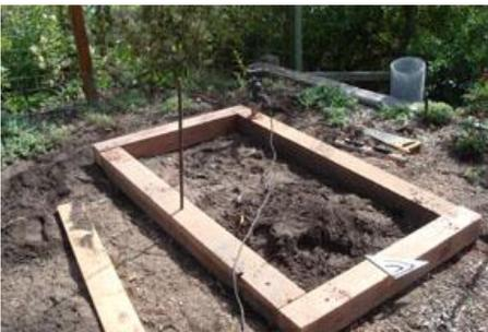
3. Set the lumber on level ground matching up the corners to make the border of the bed. Drill the holes all the way through the lumber to set the steel posts all the way through. The stakes will secure the lumber to the ground. With the mallet, pound the stakes through the wood and into the ground until the top of the post is flush with the wood.
