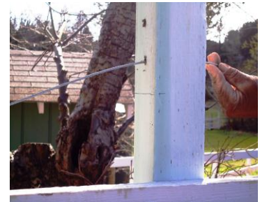
3. Thread the galvanized cable through the 1/2 inch holes in the posts.
