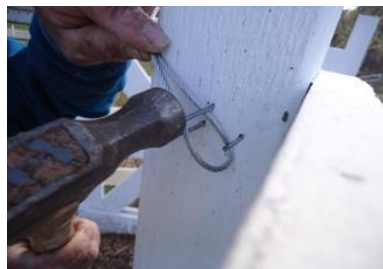
3. Secure the cable at the ends with 1 inch poultry staples.
