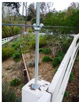
2. Wing nuts are threaded onto the rod at 10 in. apart. The galvanized cable is strung along each rod and held up by the wing
