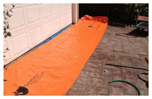
Tip: Take time to carefully place the barrier in the desired position. Once the barrier begins to fill it will quickly become heavy and difficult to move.
