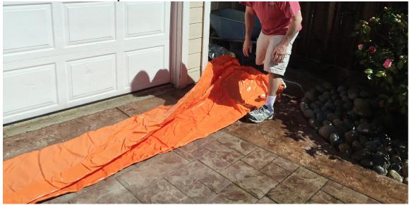
*Tip:* Take time to carefully place the barrier in the desired position. Once the barrier begins to fill it will quickly become heavy and difficult to move.
