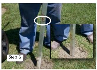
**drawn on your stake.** Next fill the hollow tube of the stake with cement. To settle the cement in the tube gently tap the sides of the stake. Finish by sloping the concrete at the base of the stake away from the ground stake so water will not puddle against it.
