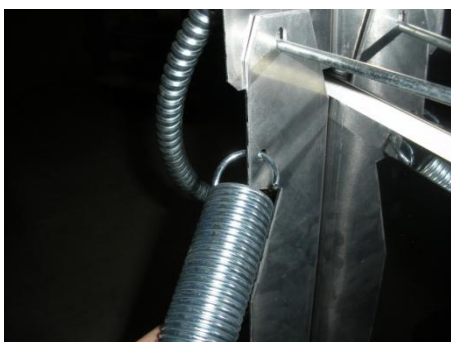
Insert the end of one spring, from the outside of the hole as shown.
