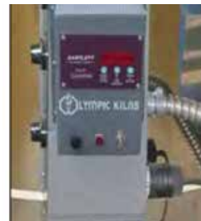
Install electrical box back on kiln with Electro Sitter installed.
