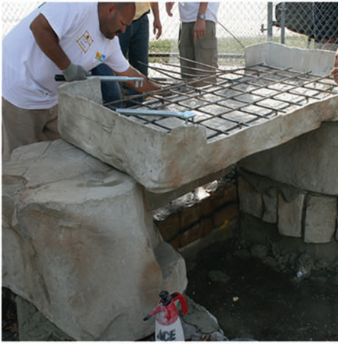
Set grotto bottom piece #6 Should be level from side to side.
