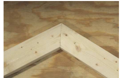
(118) Align the rafters as shown, then move to next step.
