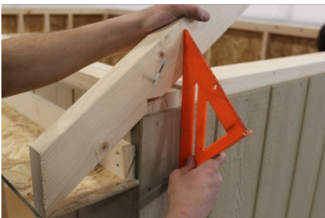
(122) Screw rafter to top plate, using a 3" screw, making sure rafter is flush with the wall siding. Repeat for opposite end of rafter.
