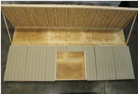
(74) Lay out siding as shown here, with the over lap towards the right.
