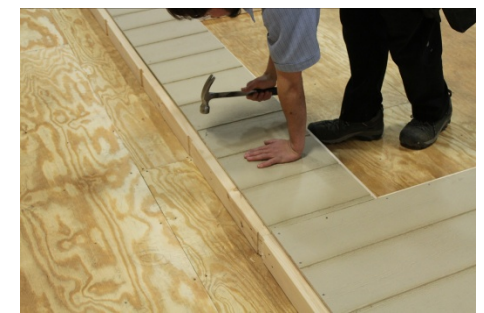
(79) Finish nailing the rest of the siding pieces above the door.
