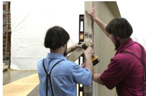
(66) Make sure the wall is level, then fasten the brace to the wall.
