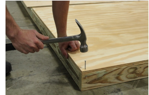
(24) Attach the corner of the flooring, using 2" nails.
