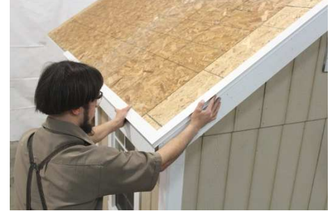
(208) Overlap the gable piece over the bottom piece and nail only the bottom.
