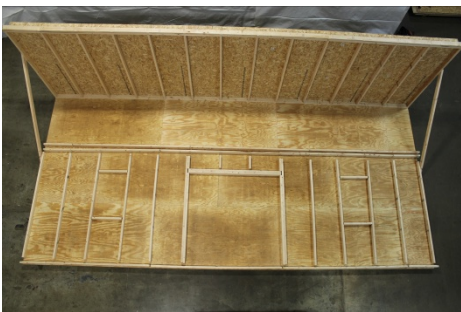
(68) Locate and lay out the parts to assemble the front wall.
