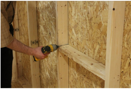
(107) Run a 2" screw through siding at each corner of the window.
