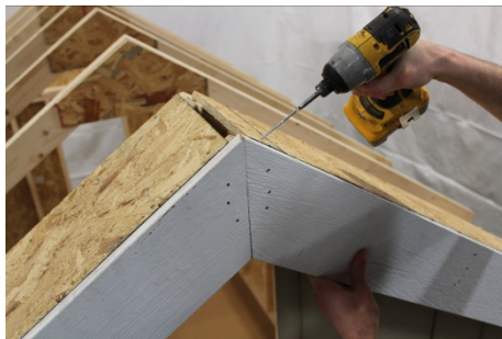
(137) Correct! Fasten firmly, using a 3" screw.
