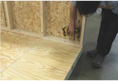
(62) Fasten to floor, using two 3” screws at every stud, trying to hit the floor joists.
