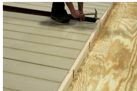
(48) Nail along the top as done in previous piece.
