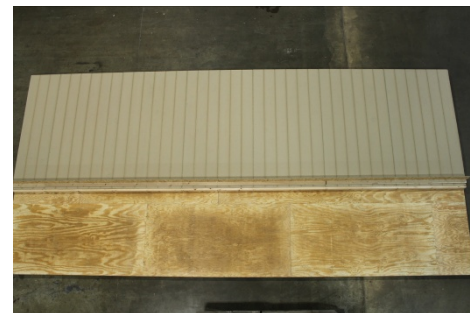
(50) Repeat previous steps for the rest of the siding.
