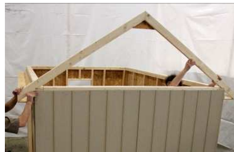
(123) Repeat these steps for the other gable rafter.
