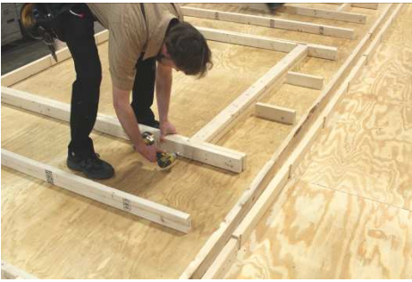
(71) Fasten both door studs with dados, to the door header, using four 3" screws.
