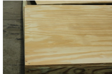
(23) Start on the front left corner with a full 4'x8' piece, making sure flooring is flush with floor joists.
