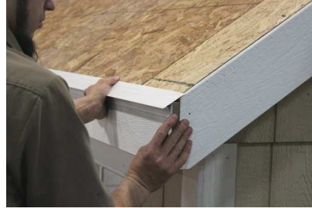
(207) Keep drip edge flush with the gable as shown, then nail every 12 to 14 inches, using roofing nails. (Nails not included.) Repeat for the next piece, keeping flush with the other gable.
