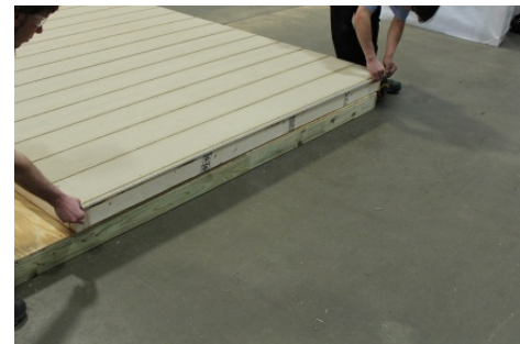
(51) Snap a line, even with the edge of the wall frame, then move to next step.
