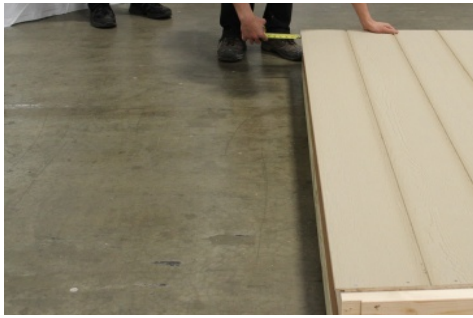
(45) Nail along the end, making sure siding is 1/2" out over the wall stud.
