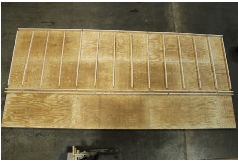
(35) Be sure to alternate the double, top wall plate splices.
