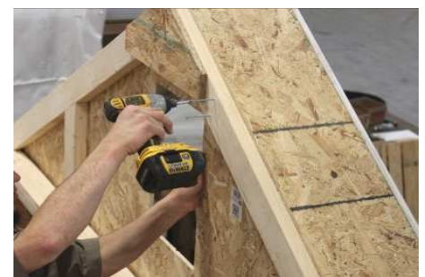
(139) Properly secure gable overhangs with 3" screws, every 10 to 12 inches.
