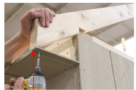
(121) Align rafter flush with edge of soffit, then screw soffit to rafter, using 2" screws. Repeat for opposite end of rafter.
