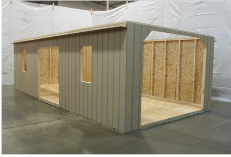
(116) Ready for rafters!
