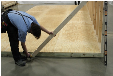
(65) Locate a rafter to use for bracing. Fasten the bottom, using two 3” screws.
