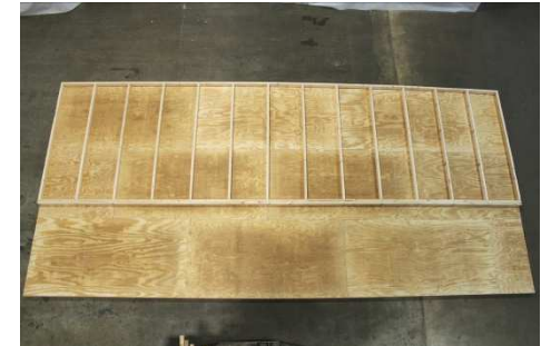
(40) Attach top plate, using 3" screws.
