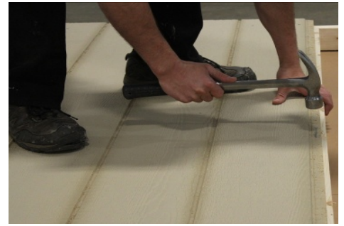
(46) Ensure that stud is parallel with siding, before nailing. Then firmly attach siding section along all edges and into each wall stud, using an 8" to 12" nail spacing.
