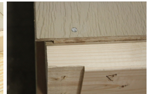
(43) Nail this corner with one 2" nail, before moving to the next step.
