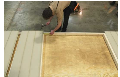
(76) Nail the bottom, again; making sure siding has 3/4" reveal along edge of door frame, then finish nailing this piece.
