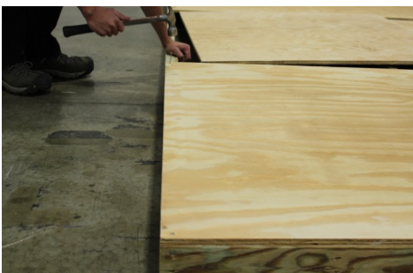
(25) Nail along the gable, again; making sure flooring is flush with the floor joist. Use an 8" to 12" nail spacing.
