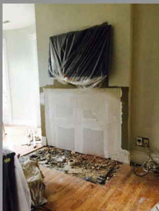
REMOVING THE EXISTING FIREPLACE
