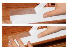
**4.** Verify that front edge of No-*Slip* Tape is aligned with front edge of step and then press the exposed adhesive onto stair surface as shown above.
