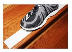
**3.** Place a foot on left side of No-*Slip* Tape, roll back the left edge of No-*Slip* Tape, and peel a small portion of backing paper to expose adhesive.
