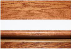
**2.** Place No-*Slip* Tape at about 1/2" from edge of step as shown above. There should be equal clearance on the right and left sides of No-*Slip* Tape. Non-*Slip* material should be facing upward.
