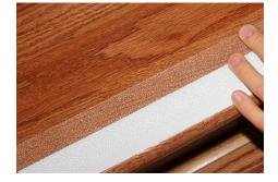
**5.** Keep No-*Slip* Tape aligned with front edge of step, then peel remaining release liner on the right half of No-*Slip* Tape, while at the same time pressing exposed adhesive onto stair surface.
