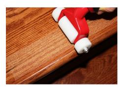
**5.** Press a roller against No-*Slip* Tape to activate adhesive and remove any air pockets. Rolling will also permit the sub-surface color to transmit through our "Clear" No-*Slip* Tape and create near-transparency.
