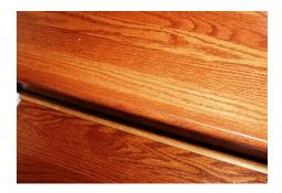
**1.** Clean stair surface — surface must be free from dirt and oils. Use rubbing alcohol to clean surface. The alcohol will remove any oils and give you a clean dry surface in minutes. Important: Make sure that the surface is completely dry before proceeding.
