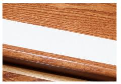
**2.** Place No-*Slip* Tape at edge of step as shown above. There should be equal clearance on the right and left sides of No-*Slip* Tape. Non-*Slip* material should face upward.
