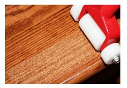
**7.** Press a roller against No-*Slip* Tape to activate adhesive and remove any air pockets if any. Rolling will also permit the subsurface color to transmit through the No-*Slip* Tape and create near-transparency.
