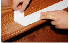
**4.** Press exposed adhesive onto stair tread while maintaining No-*Slip* Tape alignment at about 1/2" from edge of step. Continue until all backing paper is removed.
