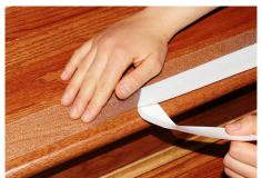
**6.** Return to left side of No-*Slip* Tape and slowly peel remaining release liner which is on the left half of No-*Slip* Tape. Press exposed adhesive onto stair surface.
