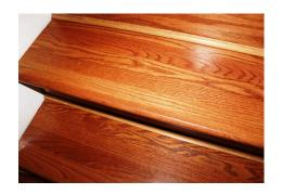
**1.** Clean stair surface — surface must be free from dirt and oils. Use rubbing alcohol to clean surface. The alcohol will remove any oils and give you a clean dry surface in minutes. It is very important that the surface is completely dry.
