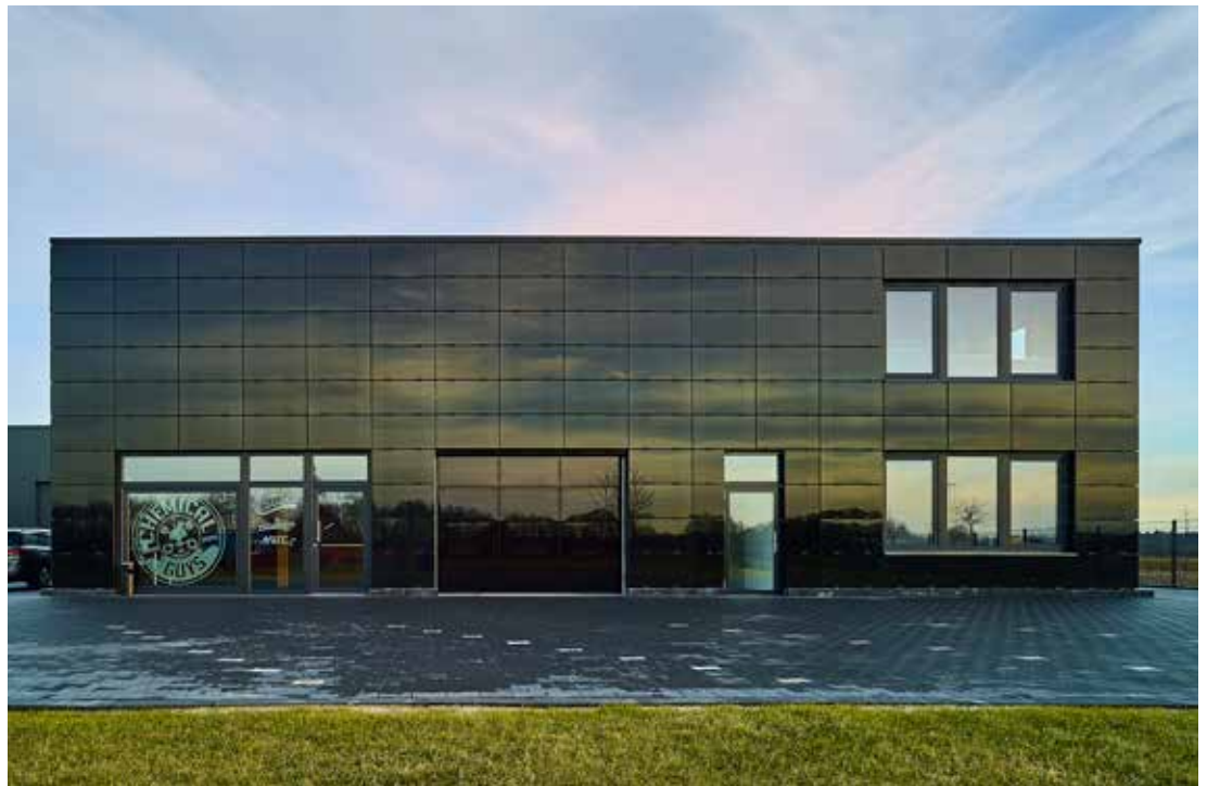
TOP. ALR F42 with on-site flush-fitting cladding made of aluminium compound boards
