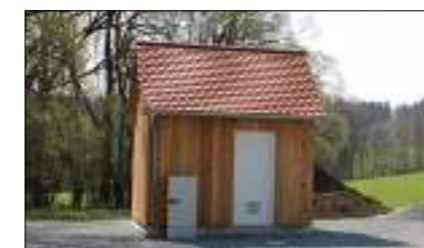
Example: Installation in a machine house
