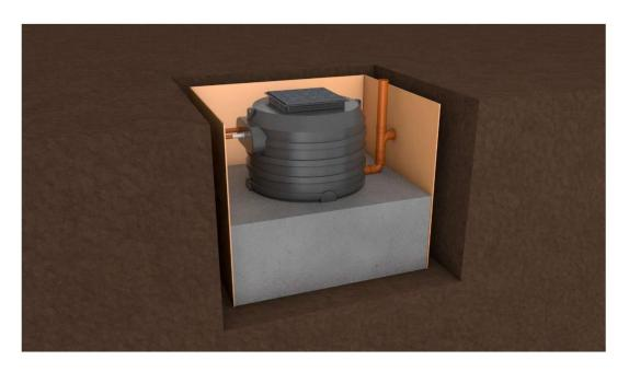
12.17. During concrete pour, ensure that tank is vertical (by use of a spirit level across the tank's opening). Additionally, ensure that the tank is at the correct depth Allow this concrete "Anchor" to set.
