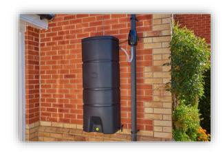
This is the installation guide for the 160L Terracottage Wall Mounted Water Butt (product code RBM-GUTWB) and applies to other terracottage products within bigger packages. This water butt weighs 10kg when empty so it is the customer's responsibility to determine, if the wall has adequate strength to support the water butt when full of water. The total weight when full and to be supported is 170kgs (a litre of water weighs approx. 1 kg).
