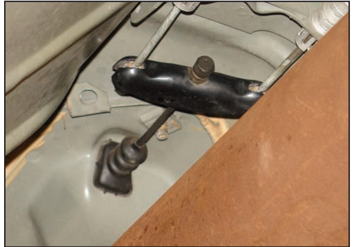
Photo 3. Installation of Cables to Balance Bar End
