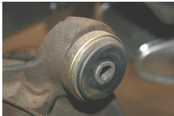
Figure 5 - Replacement Bushing Installed
