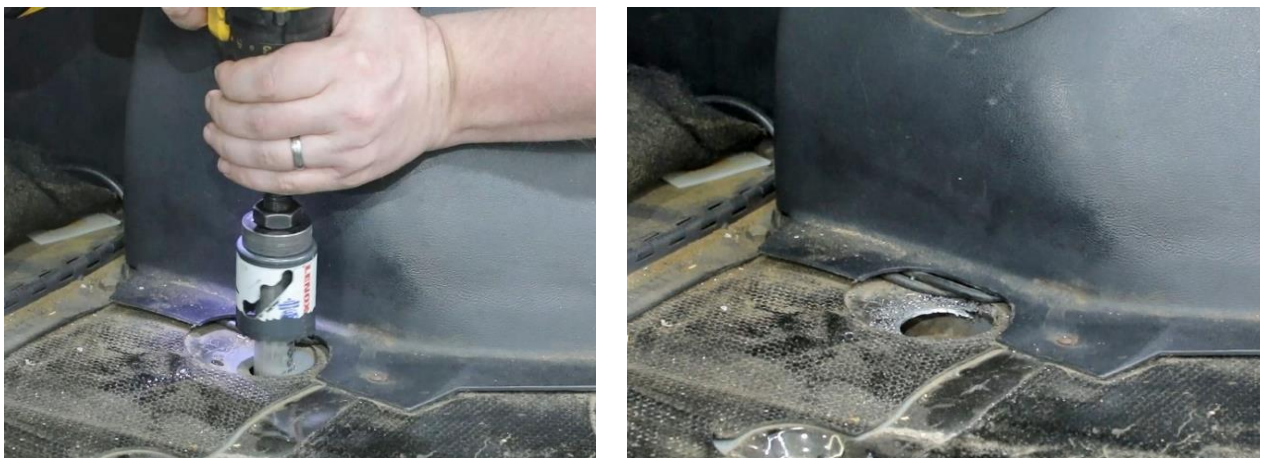
Figure 8 - Drill Access Hole
