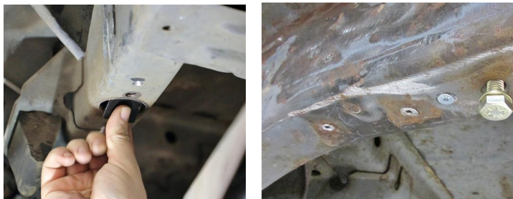
Figure 30 - Install Weld Nut Doubler Plates
