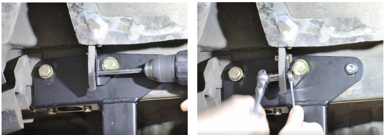
Figure 30 - Install Track Bar Reinforcement Bracket
