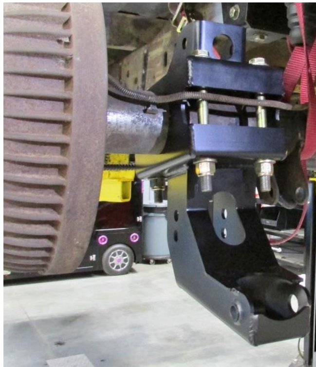
Figure 24 - Install Upper & Lower Axle Bracket (LH, Driver Side)
