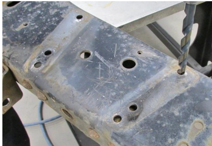
Figure 18 - Drill Out Frame Holes
