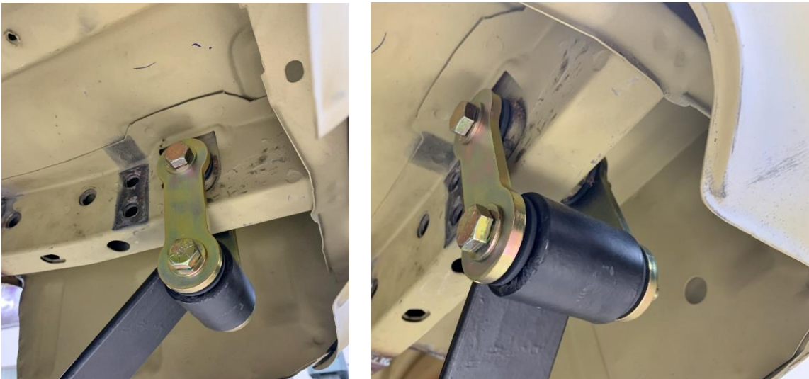
Figure 3 - Rear Leaf Spring Installed
