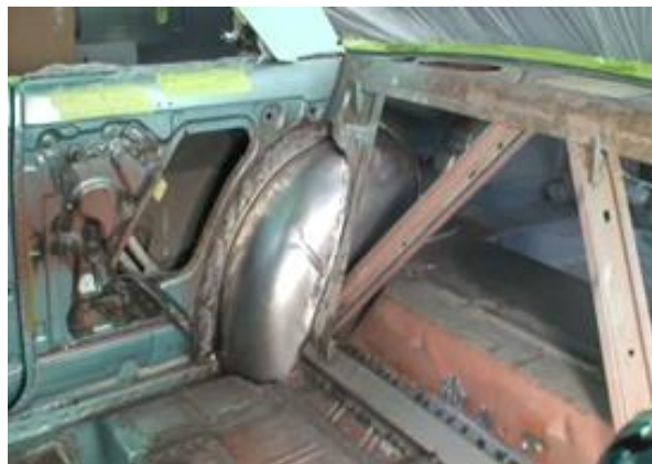
Figure 15c - Finished Modified Brace
