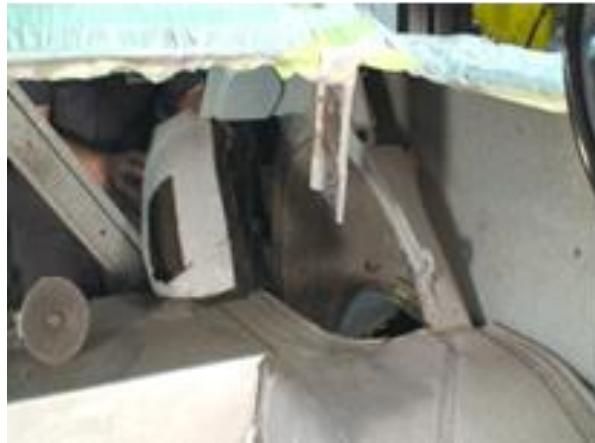
Figure 6c - Removing the Factory Wheel Well
