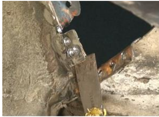
Figure 10b – Removing & Bending Lap Flange
