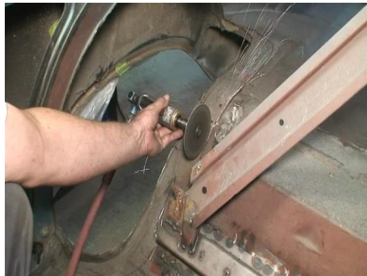
Figure 7 - Removing the Previously Traced Floor Pan Section
