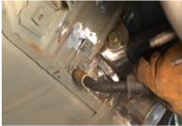
Figure 21c – Weld Anchor (Supported by Anchor Bolt)
