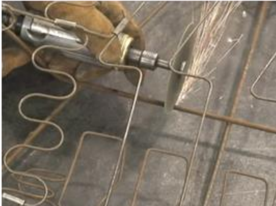
Figure 26 - Cutting the Cross Bar at the 2-1/2" Mark
