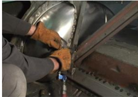
Figure 15b - Welding Modified Brace
