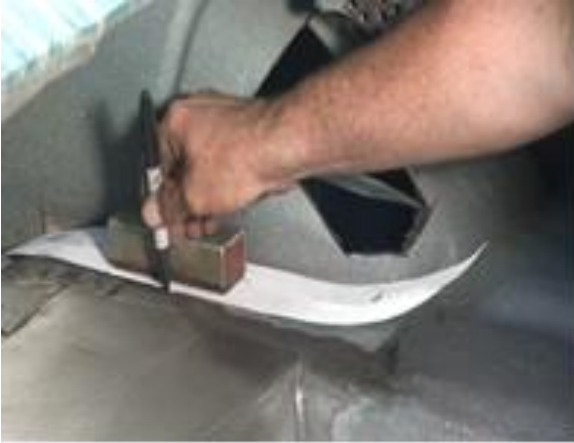
Figure 6a - Tracing the Lower Templates
