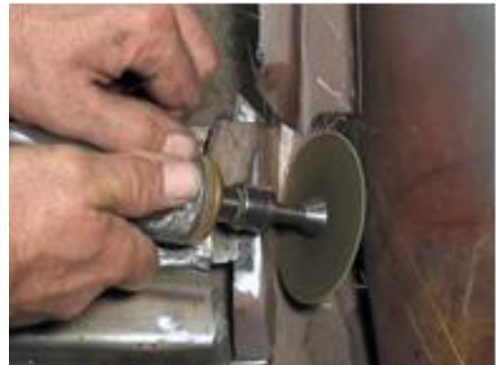
Figure 5b - Removing the Brace
